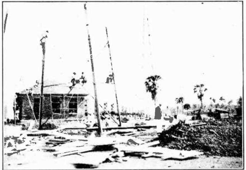
INDIA'S FIRST BROADCASTING STATION. Constructional work in progress on the Bombay Broadcasting Station, which was opened by the Viceroy on July 23rd. Bombay's call sign is 2BY; its power is 3 kW.
